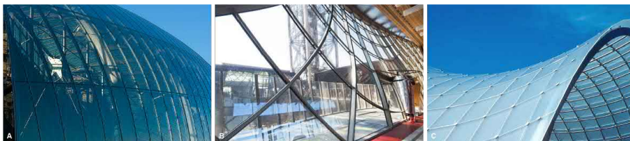
Figure 2. Double-curved facade paneling following the principal curvature directions. A: The Strasbourg train station. B: The Eiffel Tower Pavilions. C: The Schubert Club Band Shell.
